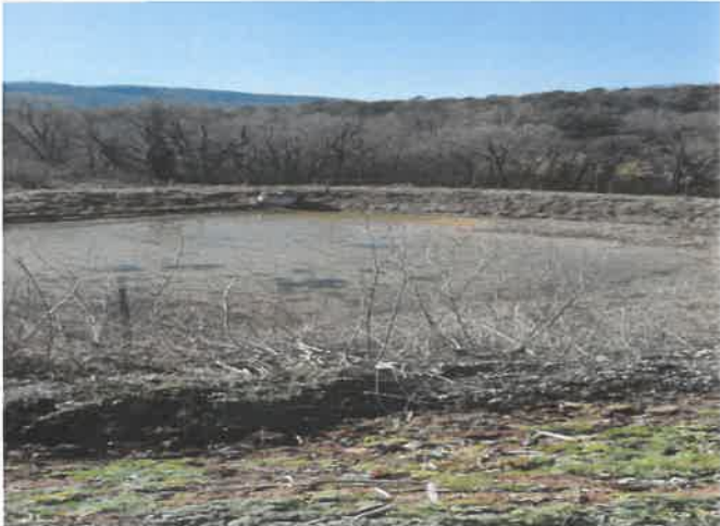
Storm water pond prior to outfall 002
